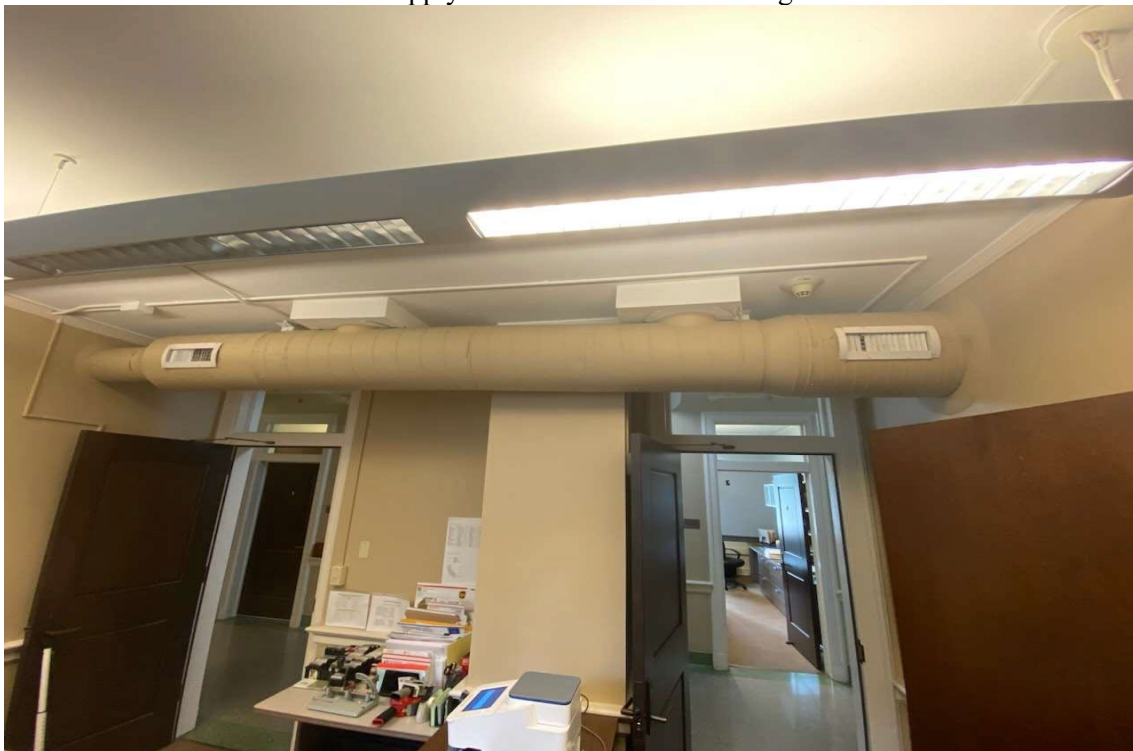
Supply Vents on Older side of Bldg.
